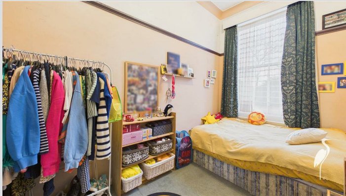
Single glazed sash window to front.
